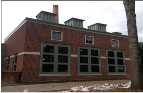
Figure 22: Co-generation heat plant located on the Keene State College campus
